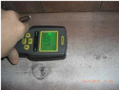
Sill plate garage side
