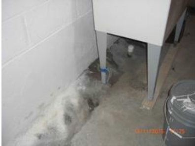
Water leak from wall
