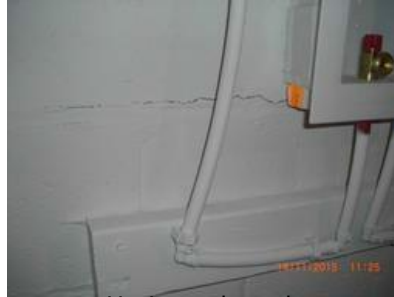
Horizontal crack
