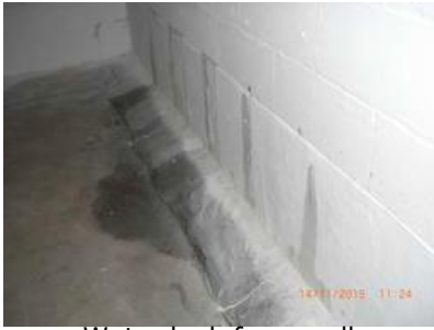
Water leak from wall
